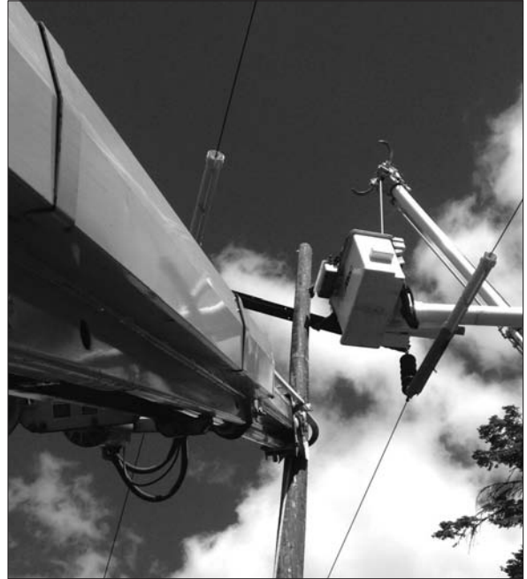
Below, the crews replaced the pole "hot," leaving all customers with power while completing their work.
